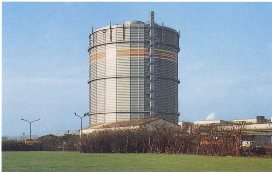
LEFFER Gas holder Type MAN approx. 100.000 cu. m. at Thyssen Stahl, Duisburg/Germany
